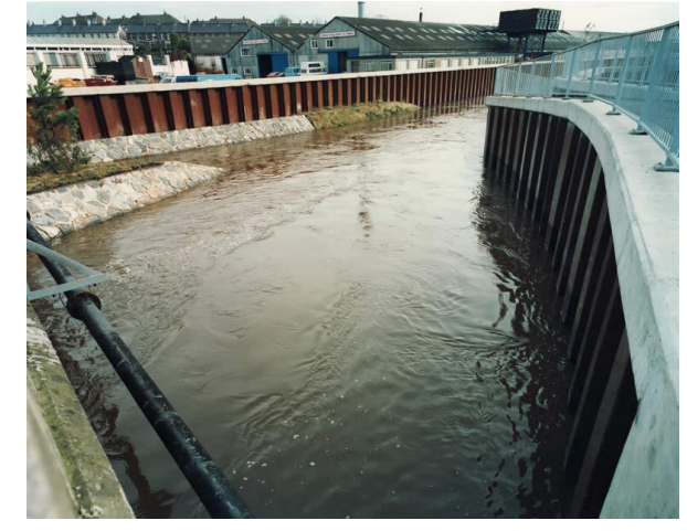
Sheet Pile Finish
