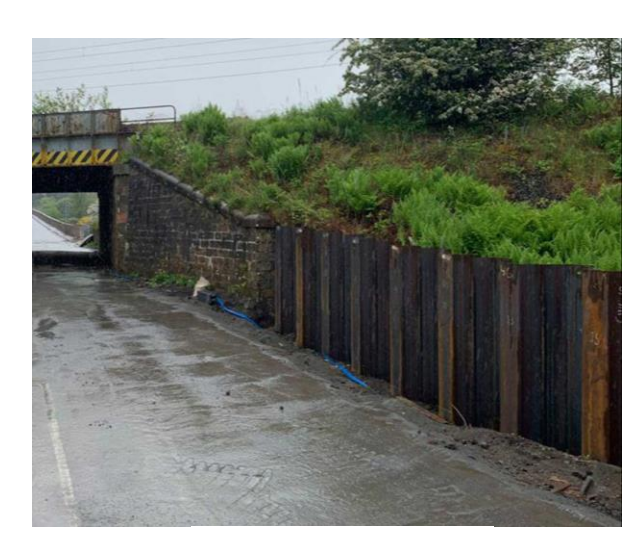
Sheet pile finish
