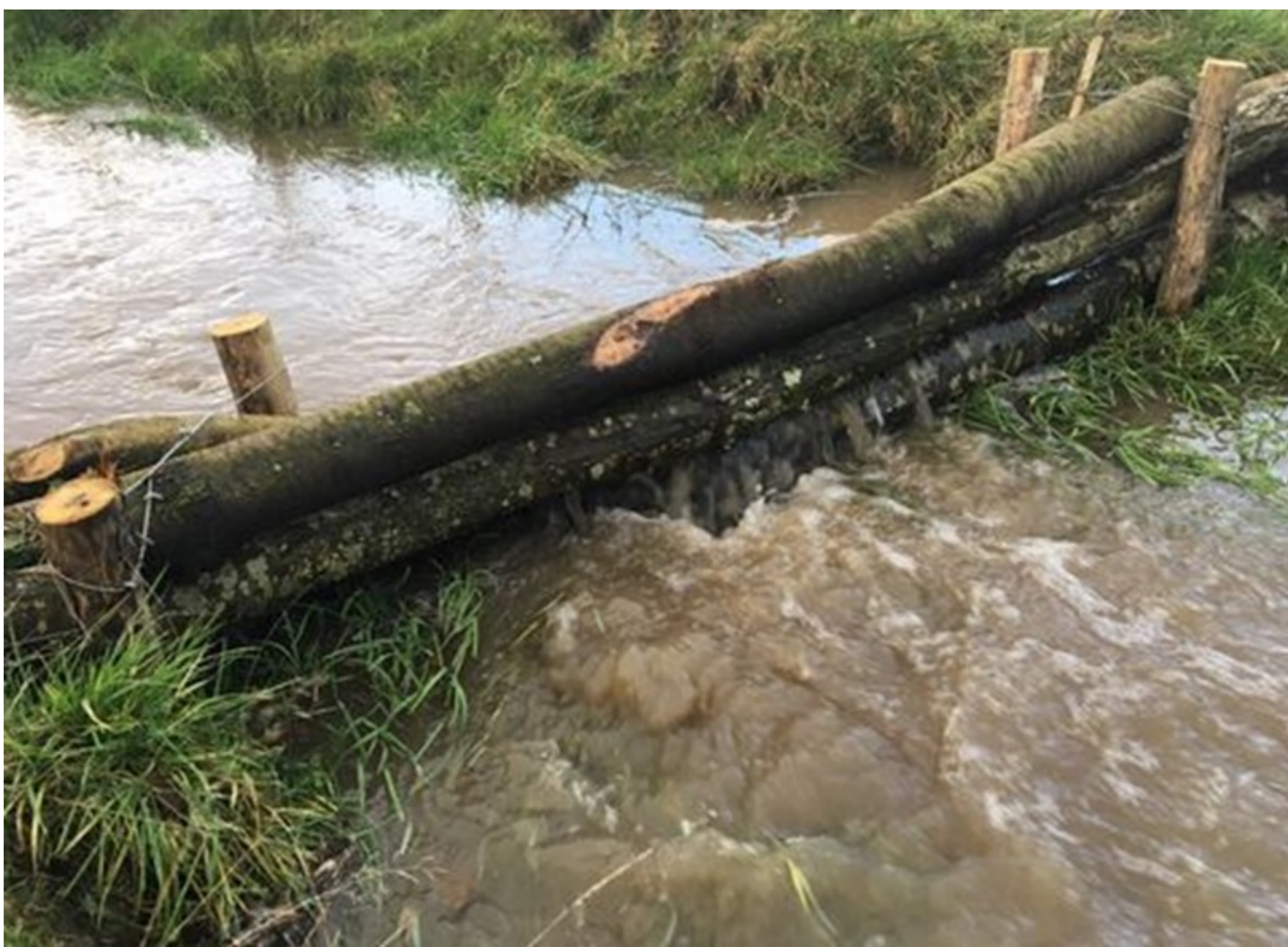
Figure 25. Example of leaky barriers (source: Warwickshire wildlife trust)
