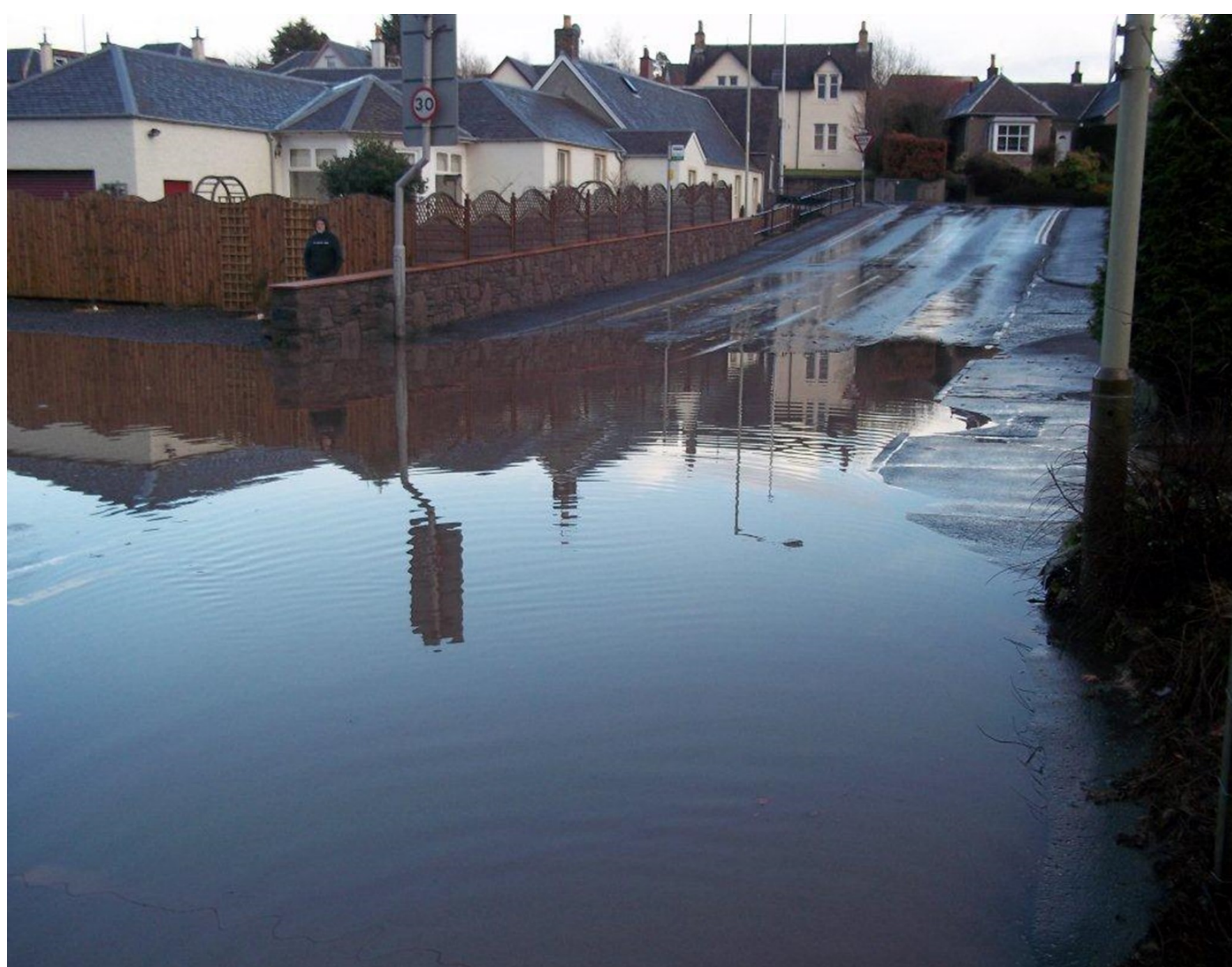
Figure 7. Flooding at Stormont Road (2024)
