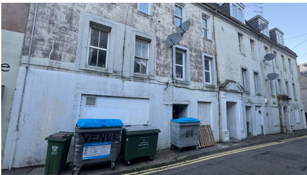
Figure 67 – Poor maintenance and lack of bin storage on Watergate
