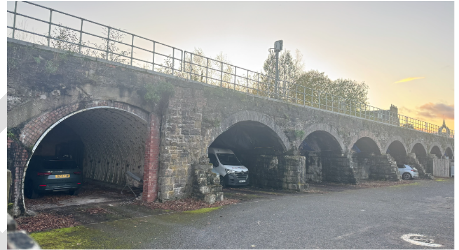
Figure 63 – Railway viaduct visible from Tay Street
