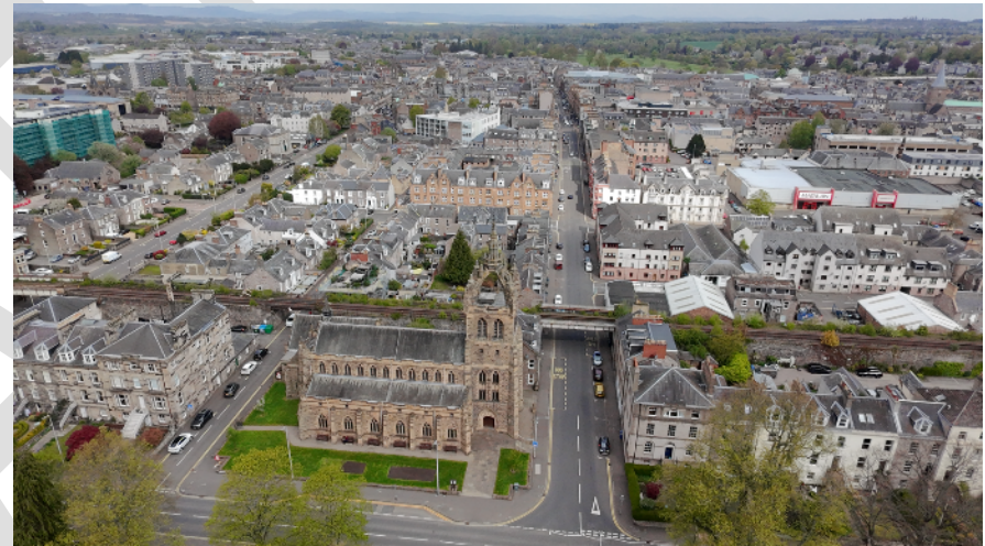
Figure 69 – St Leonard's in the Field and Marshall Place terraces
