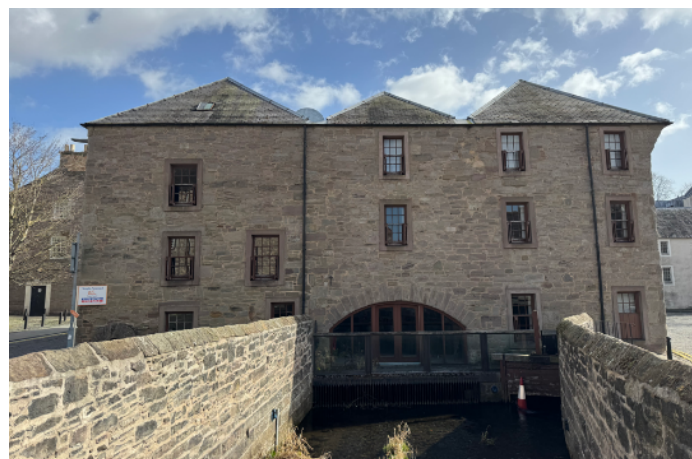
Figure 43 – The vacant Lower City Mills building
