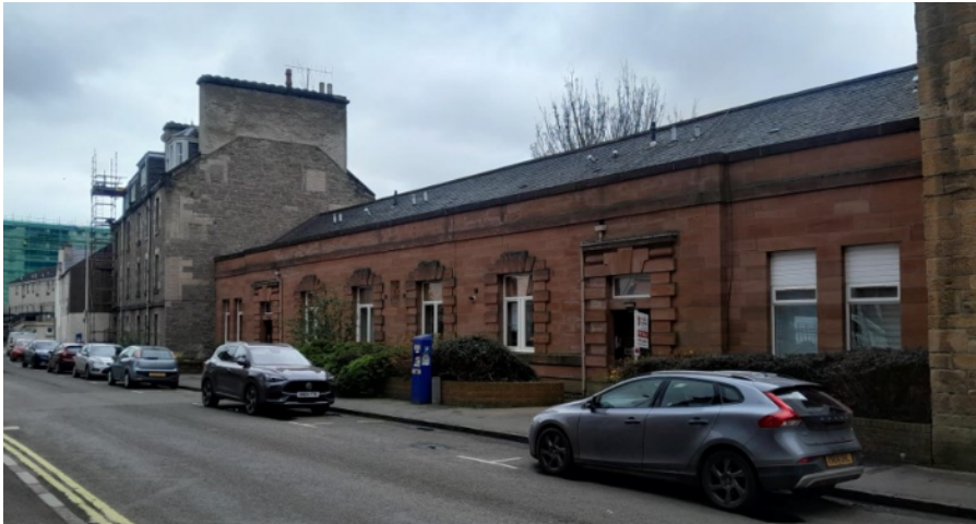
Figure 84 – Single-storey development on Alexandra Street.
