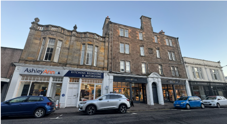
Figure 62 – Two unlisted building of merit to the right and the listed former photographic studio to the left
