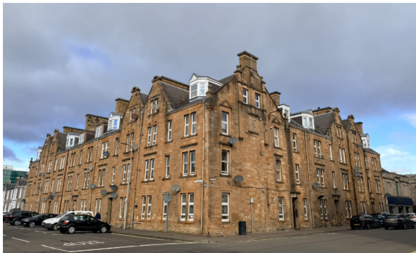
Figure 76 – Upvc windows and satellite dishes detract from the character of this building
