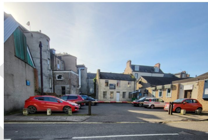
Figure 56 – West side of Barossa Street in poor condition
