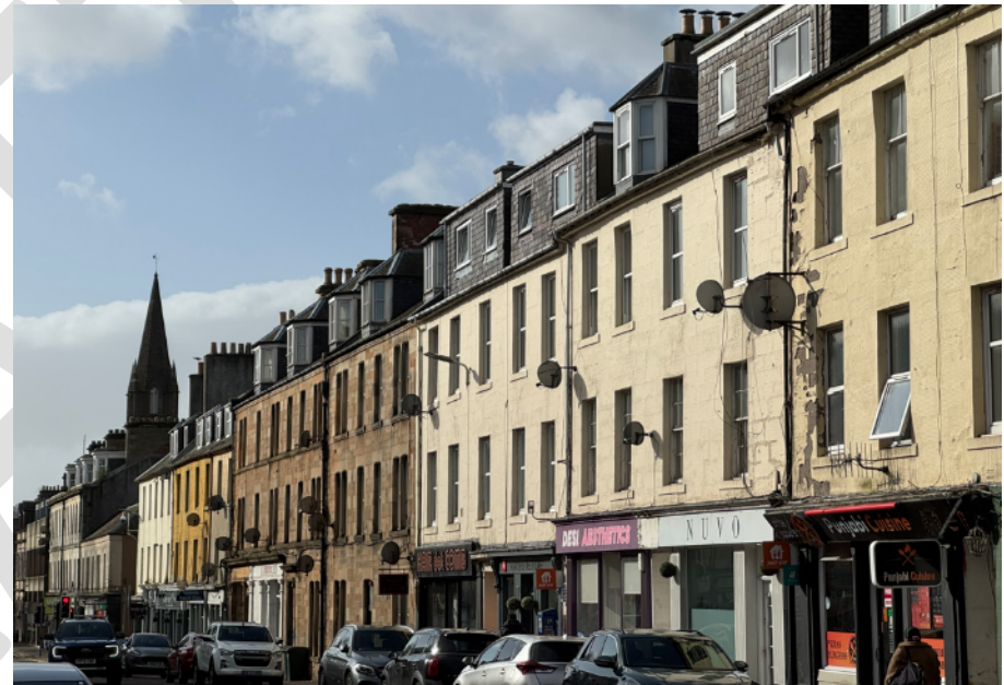
Figure 39 – St Paul's spire in views from the north along North Methven Street
