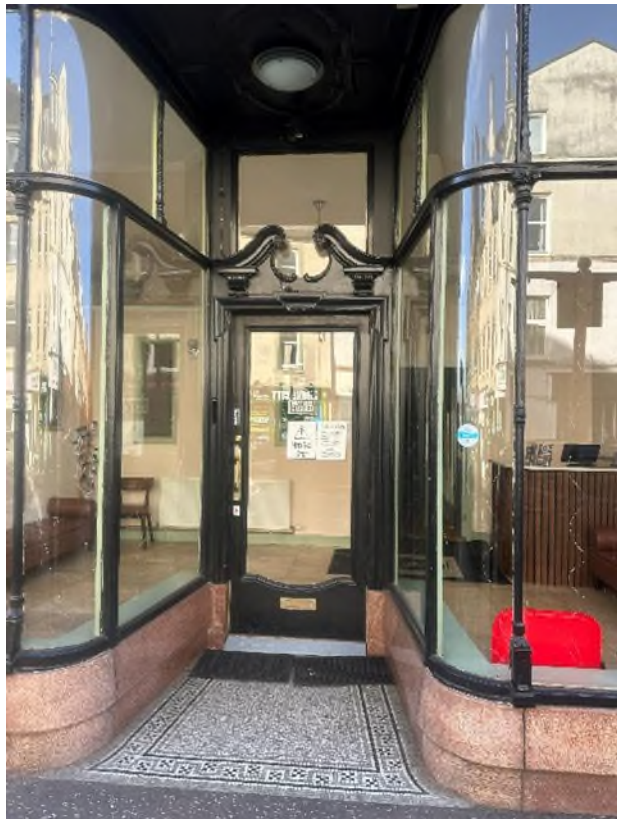
Figure 25 - Unlisted historic shop front in South Methven Street
