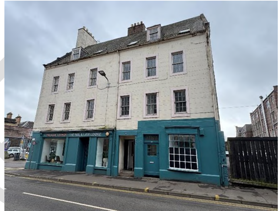
Figure 24 - Historic shopfront on the corner of South Street and Speygate
