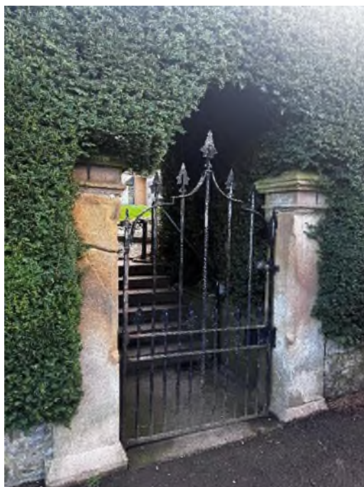
Figure 46 – Decorative stone gatepiers and iron gates at Fairmount Terrace
