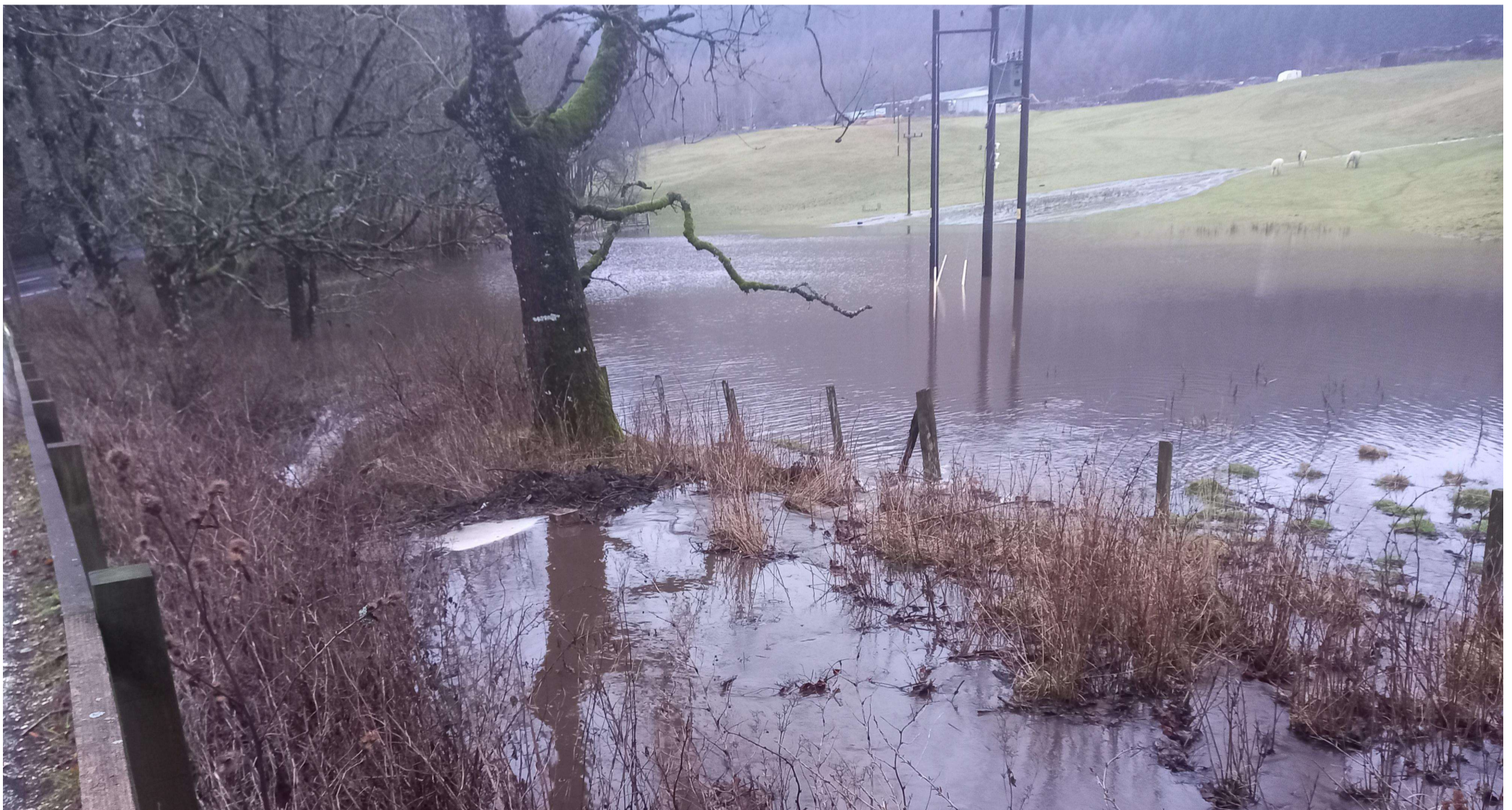
Figure 14: Natural low point North of the Kings Pass / Blairgowrie Road junction, shown to be currently subject to flooding.
