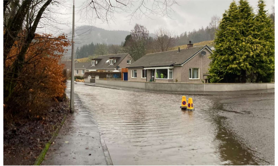
Figure 7: Flooding from burn at Atholl Gardens
