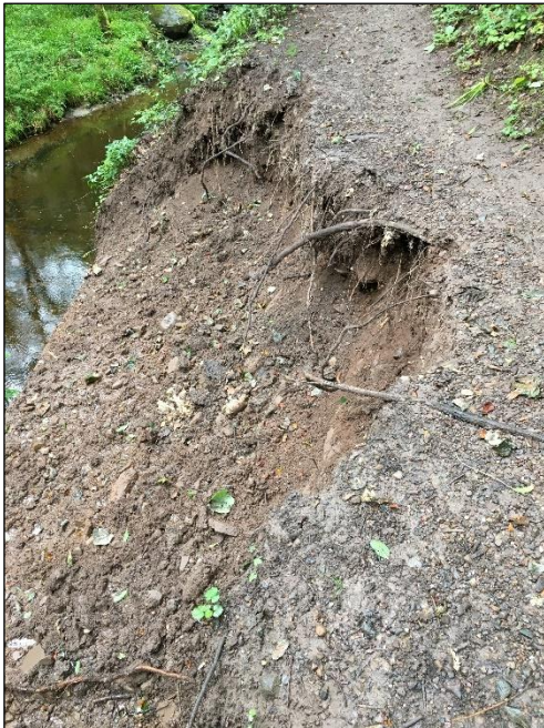
Photo: Landslip in Upper Den
