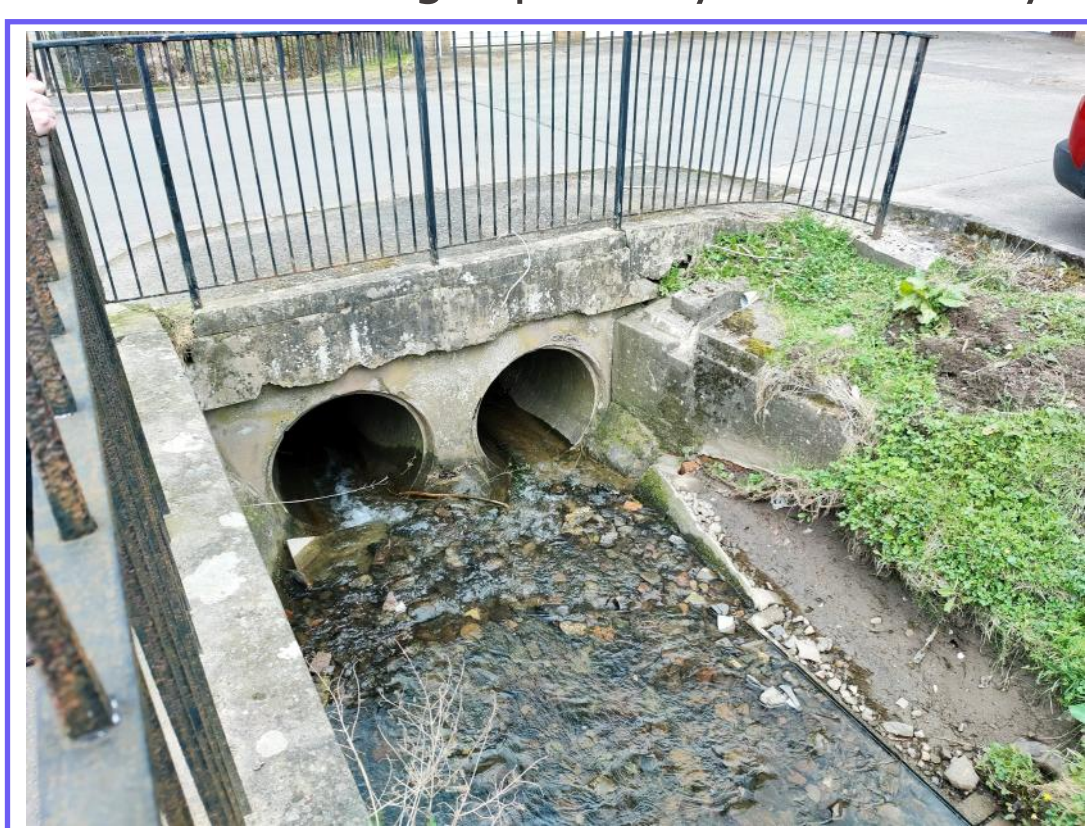
Upgrading the Culvert
