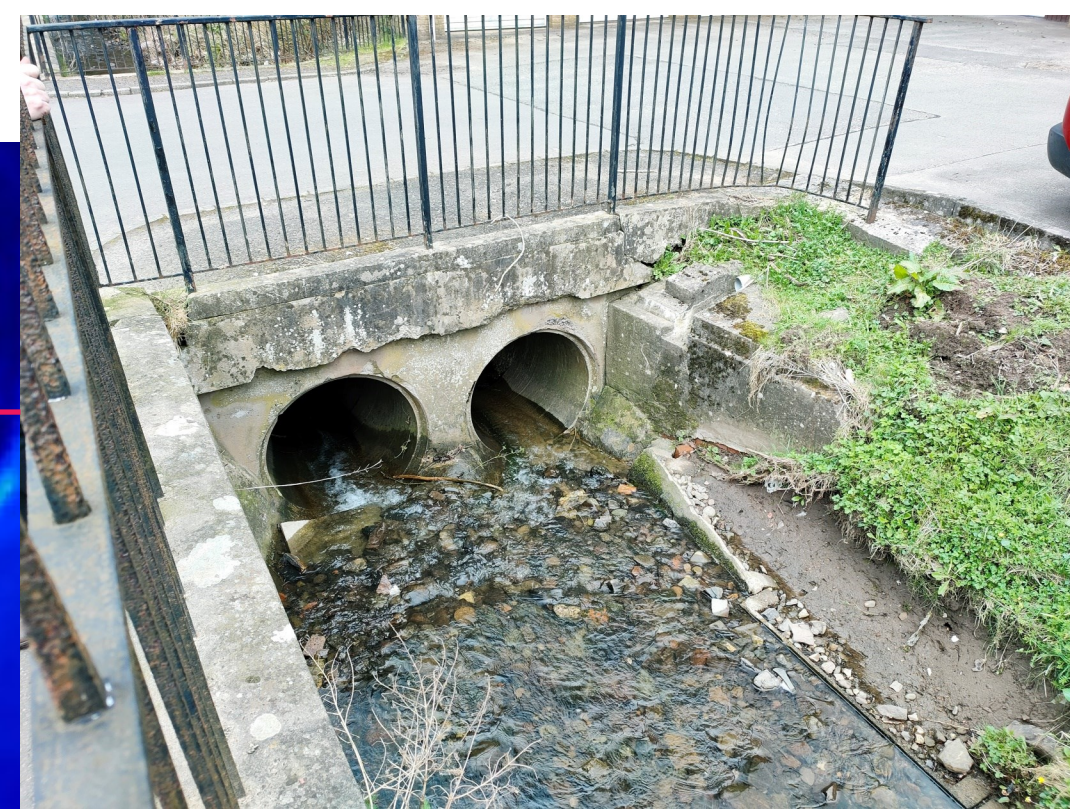
Existing Culvert at Queens Court
