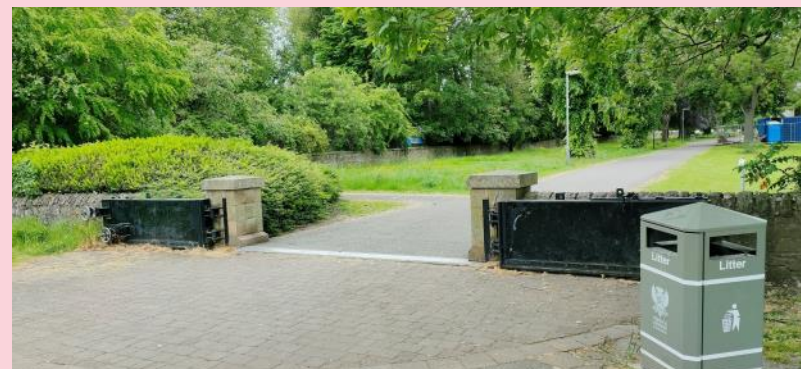
Flood Gate on South Inch, Perth
