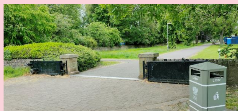
Flood Gate on South Inch, Perth
