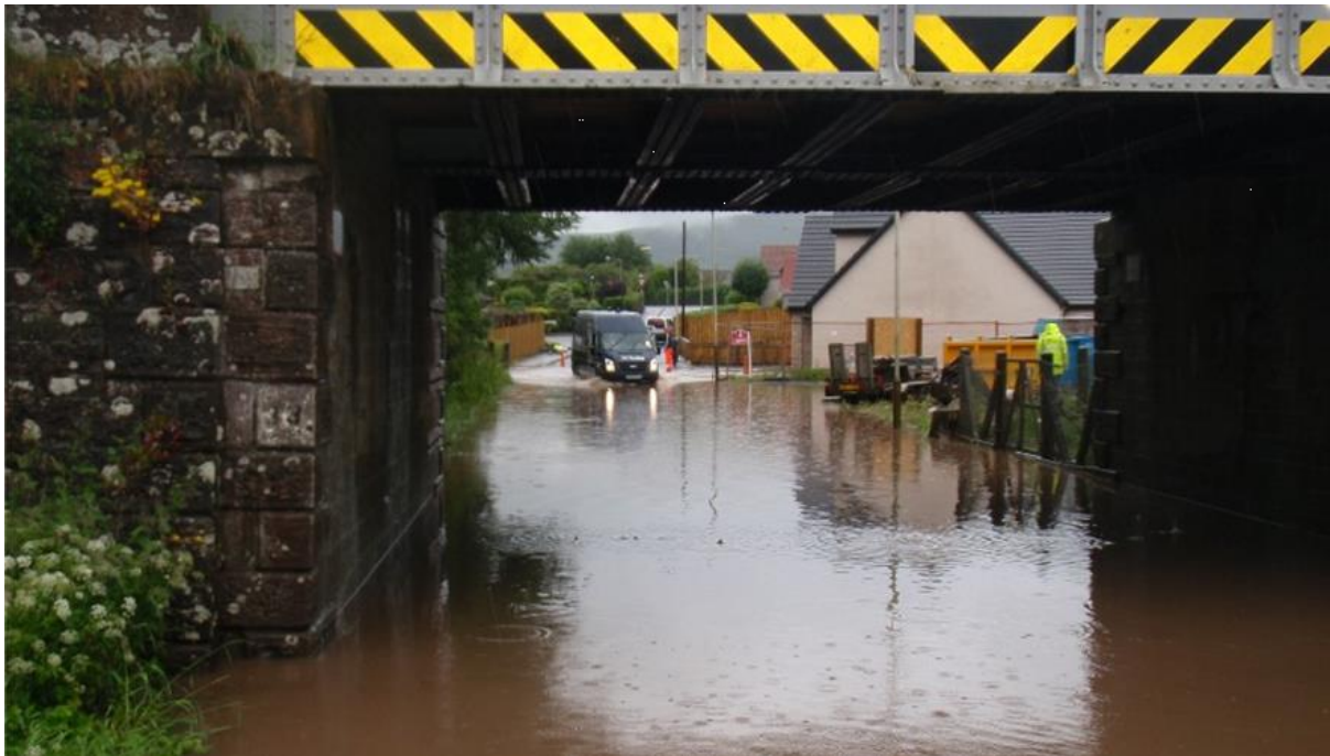
Figure 6. Flooding at Old Edinburgh Road (2012)
