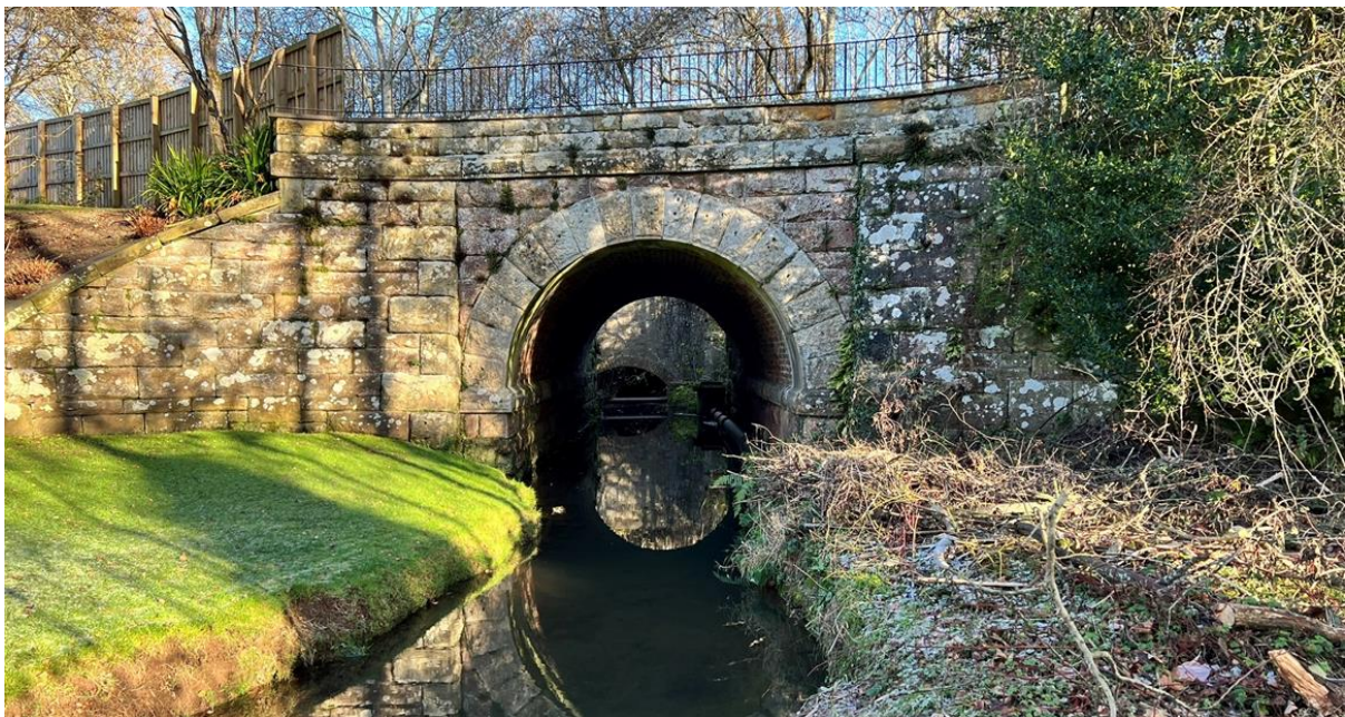
Figure 1. Deich Burn at Bridge of Earn.
