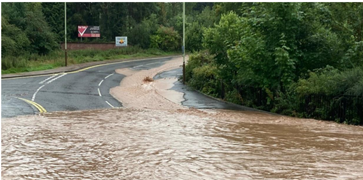
Figure 2. Example of surface water flooding.
