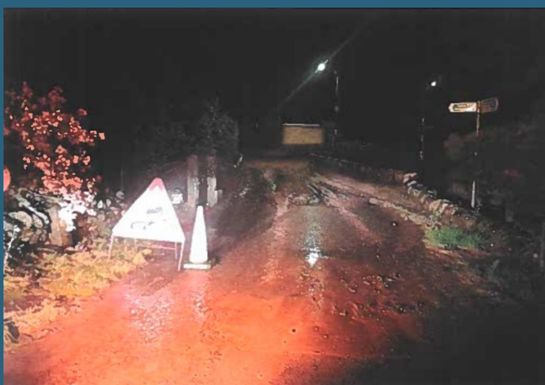
▶ Figure 7. Proposed location of speed hump, showing deposition from overland flow during the flood event of November 2023
