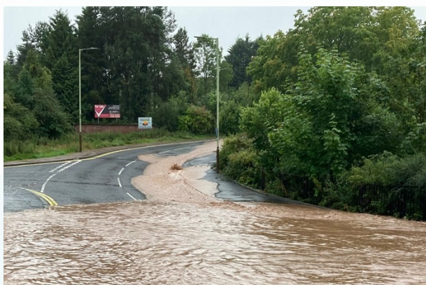
Example of surface water flooding
